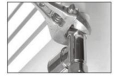
4. Insert the pipe (at this point you will have already prepared the water supply pipes to match up with the radiator or towel rail and valve dimensions). Then tighten the nut (with the olive already in place) that holds the pipe in position.
